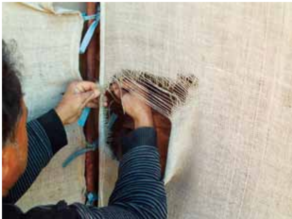
Figure 12. Patching of holes in panels.
