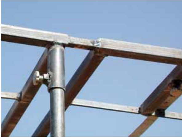
Figure 7. Detail of trellis, showing link among components.
