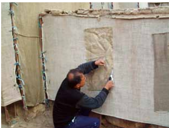
Figure 13. Patches on panels.
