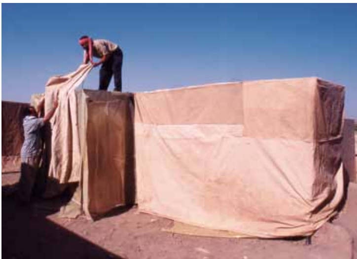
Figure 10. Tarps being draped above trellis.
