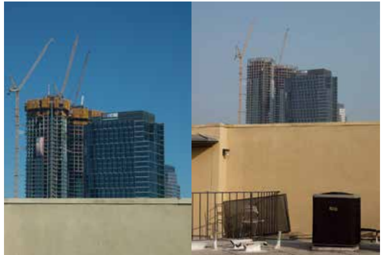
Figure 7. The luxury condominium building Century Plaza goes up near the intersection of Constellation Boulevard and Avenue of the Stars. Left: My view on July 4, 2020, with a celebratory five-story Stars and Stripes and the working platforms and third crane still in place. Right: Two months later, the concrete skeleton of the top floors is finished and the working platforms and third crane have been removed.
